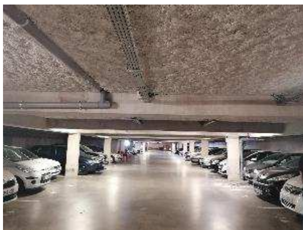
Structure poteaux-poutres parking
